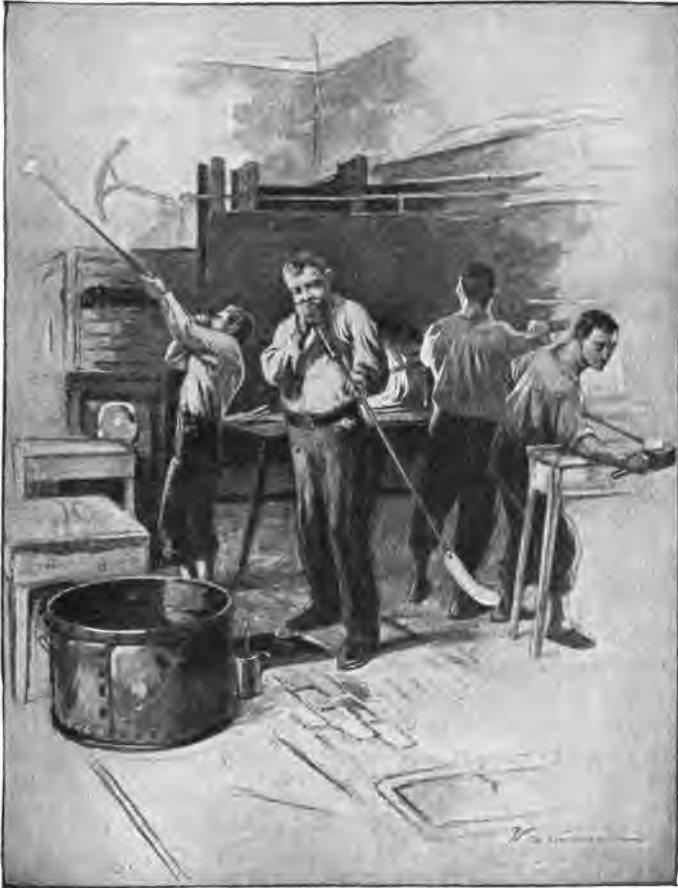
FIG. 88.—Various steps in glass blowing.
